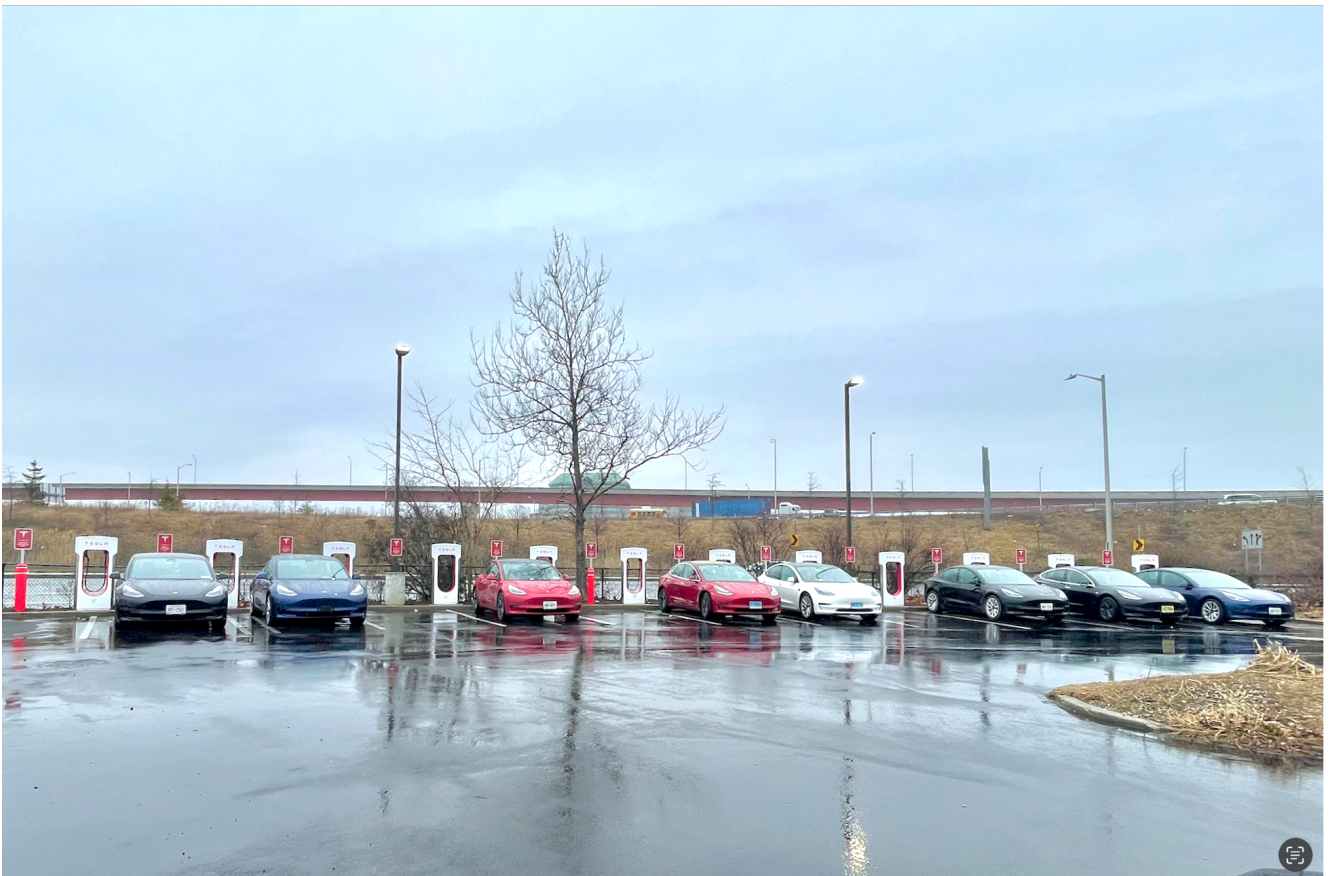
Hotel Marcel New Haven Superchargers with Teslas
