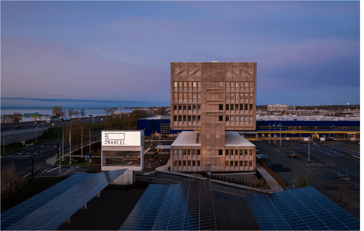
Hotel Marcel, formerly Pirelli Tires HQ, with solar canopies in foreground.
